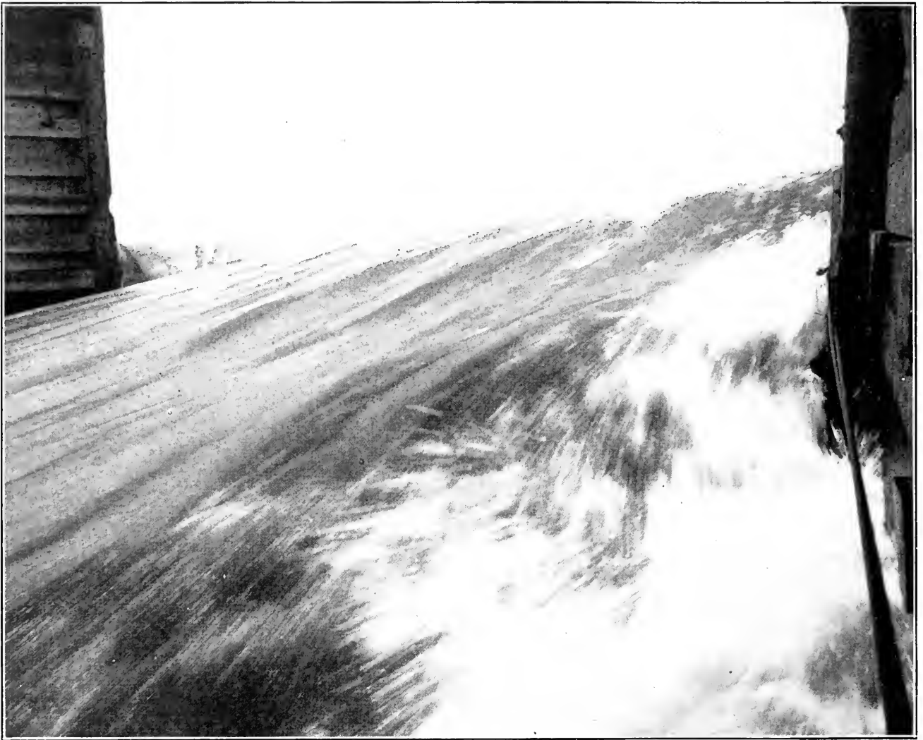
THE GAP BETWEEN THE COFFER-DAMS
